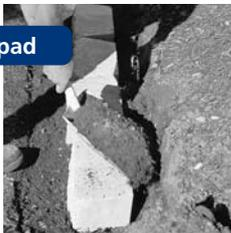
Spread road base along the bottom of your trench. When using road base, level with a straight edge and compact to the required height by tamping with the rear face of a block or mechanical whacker packer.
