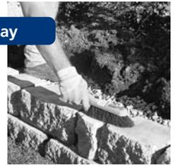
Add your subsequent block courses to your maximum height. Remember to backfill with drainage aggregate as you go, and compact it when 300mm deep. Sweep the top of each course before laying the next to remove all loose stones. Ensure the locking lips (at the back or top of the block) fit snugly together.
