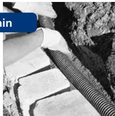
If required place a 100mm drainage pipe behind the first course of blocks on the bed of drainage aggregate. Outlet the drain through the wall at every low point, at every 20m of wall length, and around the ends of the wall to your storm water system.
