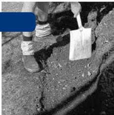
Dig a trench 300mm-600mm wide and 130mm-150mm deep to fit the leveling pad. Remove any roots and soft earth. Level and firmly compact the soil at the bottom of the trench.
