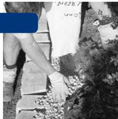
When the first course is in place, backfill behind the blocks with a minimum 300mm wide 10-20mm blue metal drainage aggregate to a level slightly lower than the block height. Lay in the second block course then backfill immediately behind the wall with the drainage aggregate.
