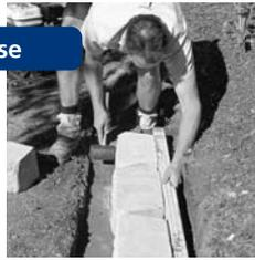
Place blocks side by side at the front of the leveled and compacted road base whilst using a string line along the back of units for alignment. For curved walls, place the blocks against the required shape formed by a garden hose and marked out with spray paint. Make sure the blocks are tightly side butted together and true to the running edge of the finished wall. Sweep the top of the first course before laying the second.
