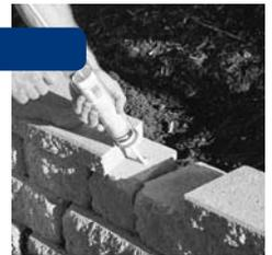
Backfill to the final wall height whilst being careful not to nudge any blocks out of alignment. Capping units should be glued to the top course using a construction adhesive. (Liquid Nails)
