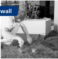
For straight walls use stakes and a string line. For curved walls set the shape by laying a garden hose on the ground, then mark the curve with spray paint. Its best to use a hose with a tap on the spray nozzle of, as the water pressure will form a more uniform curve.
